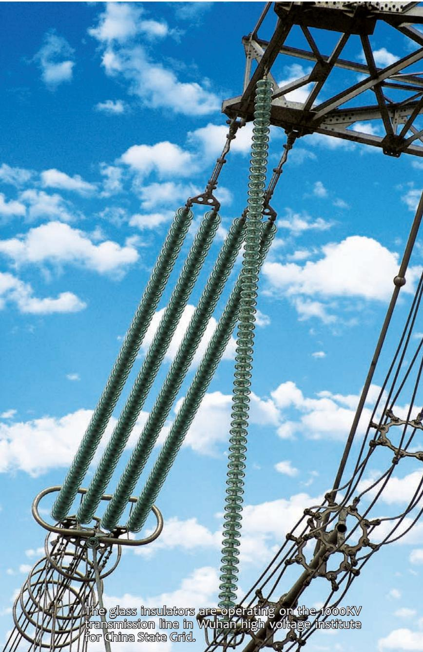
The glass insulators are operating on the 1000KV transmission line in Wuhan high voltage institute for China State Grid.
