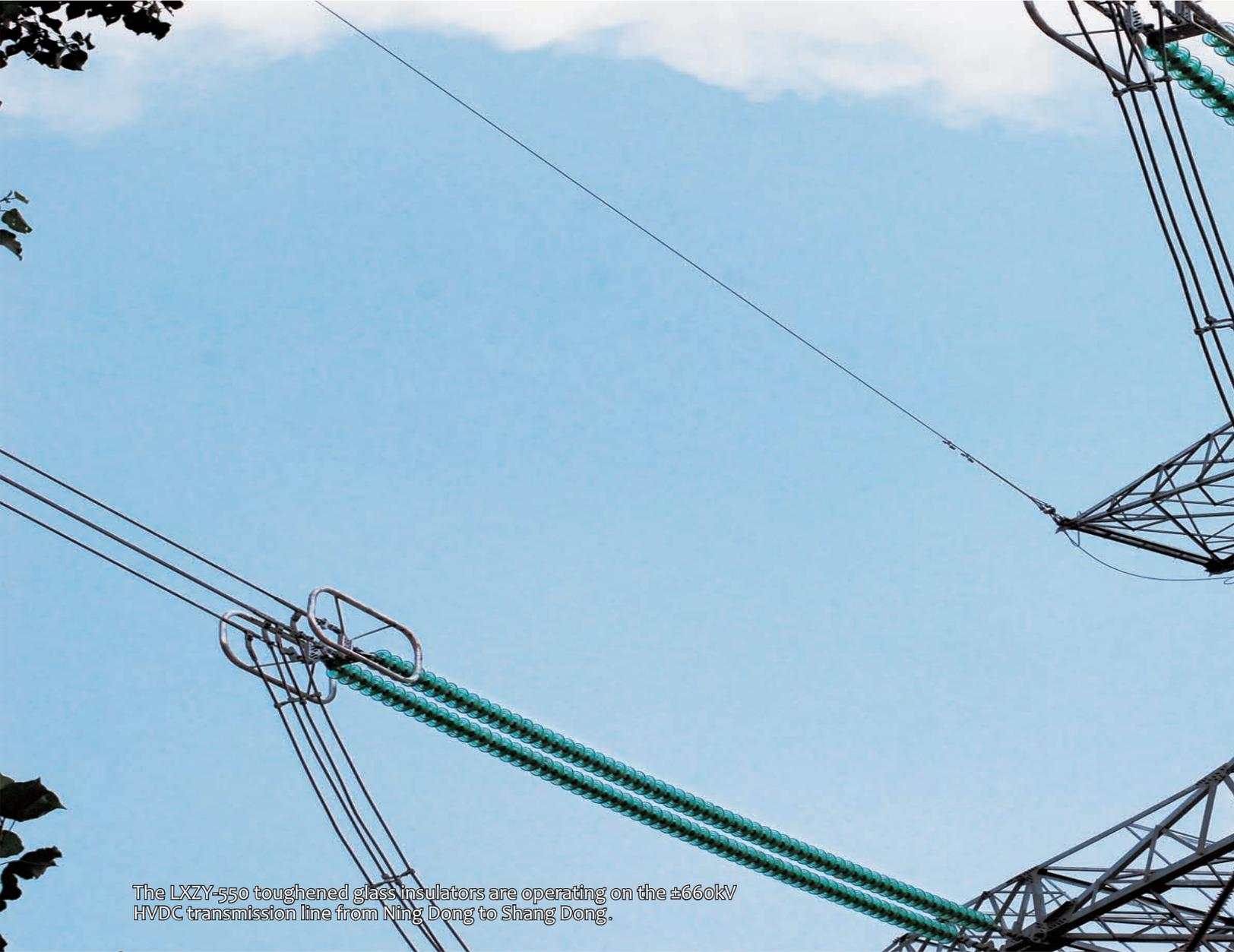
The LXZY-550 toughened glass insulators are operating on the  $\pm 660$ kV HVDC transmission line from Ning Dong to Shang Dong.
