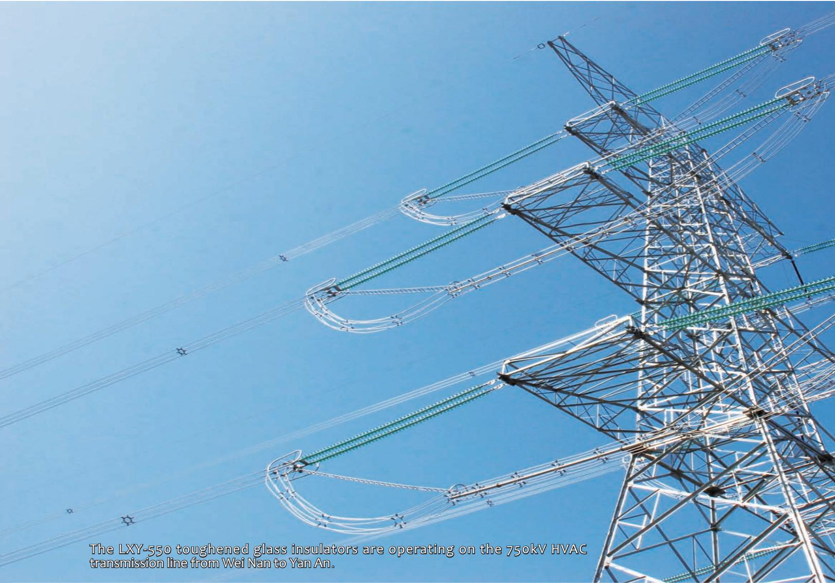
The LXY-550 toughened glass insulators are operating on the 750kV HVAC transmission line from Wei Nan to Yan An.
